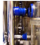
NOT properly docked
